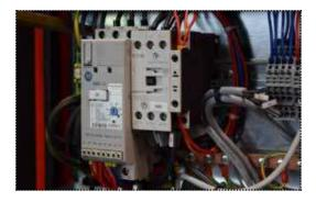
Motor **soft-starter** allows a reduction of the load and torque in the power train and electrical current surge of the motor during start-up.
